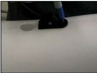
Set the lock in place approximately 1/4" below the hole. Mark the socket through the hole in the lock.
