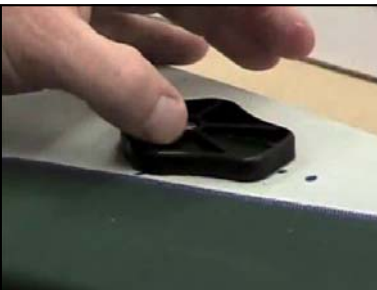
Quickly set liner attachment in marked location.
